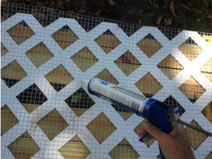
You will have to make sure you put some clamps or weights on the fence after caulking so that the caulk can adhere to the plastic lattice work and the hardware cloth.
